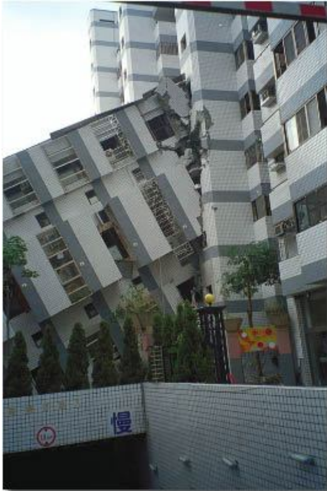
Hollow Plinth Collapse in Highrise
