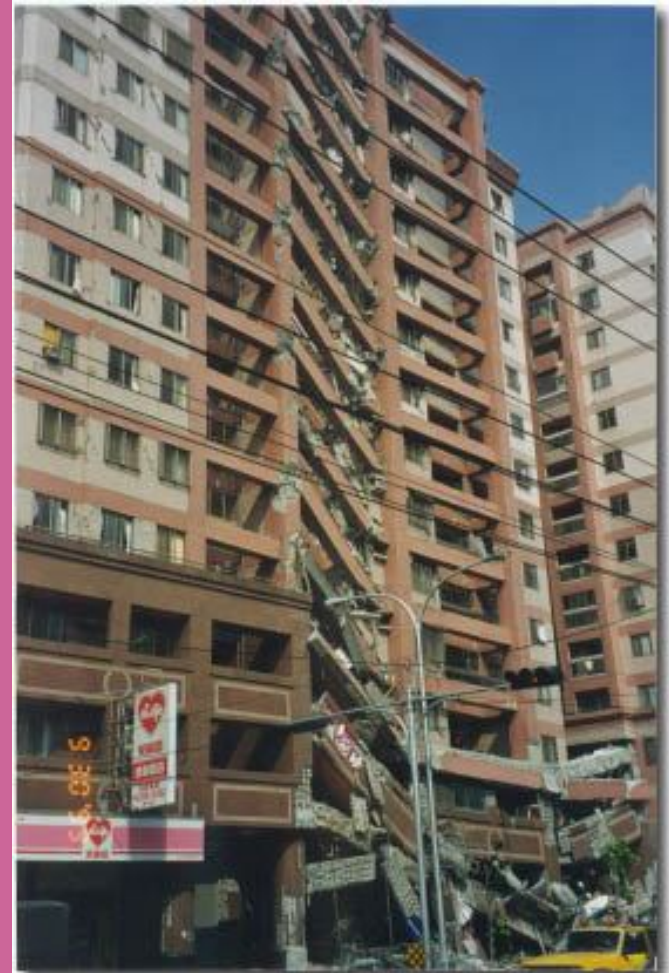
Hollow Plinth Collapse in Highrise
